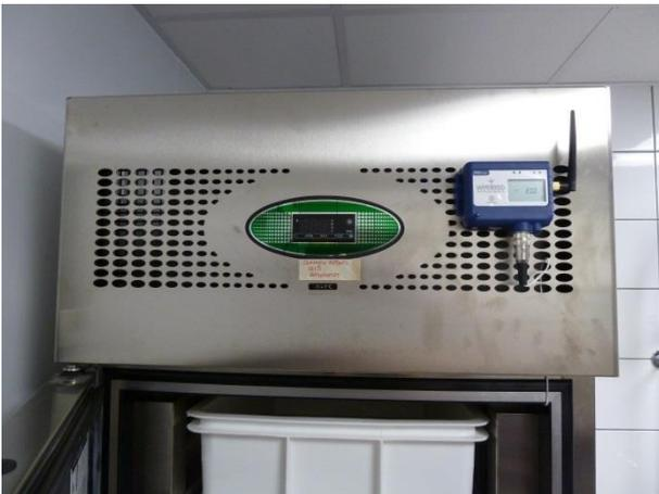
If it's not this style of fridge or freezer then use standard installation method, in certain circumstances the double sided tape will not stick to the surface of the fridge or freezer then mount Tx on top and use clips with silver masking tape to attach to the surface. (As shown in photo below)
